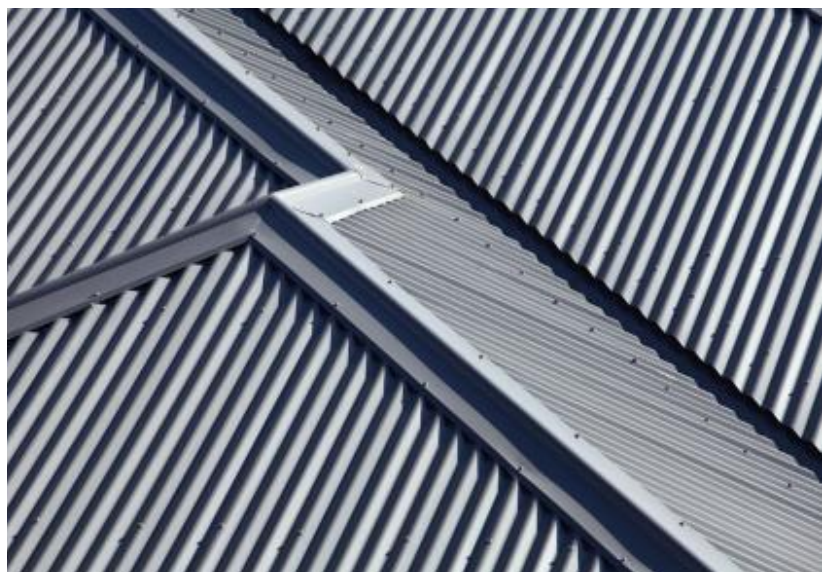
SHEET METAL ROOF
