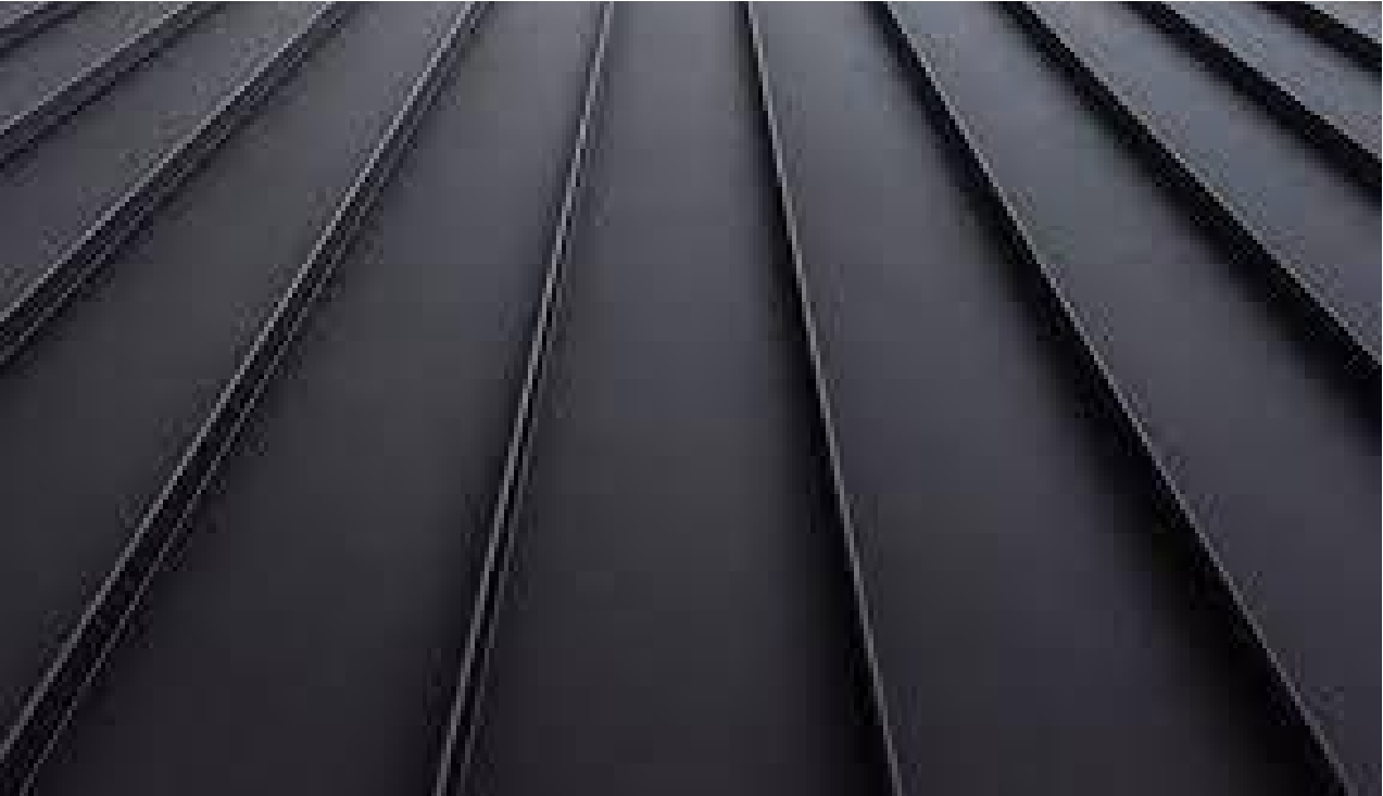
SHEET METAL ROOF
